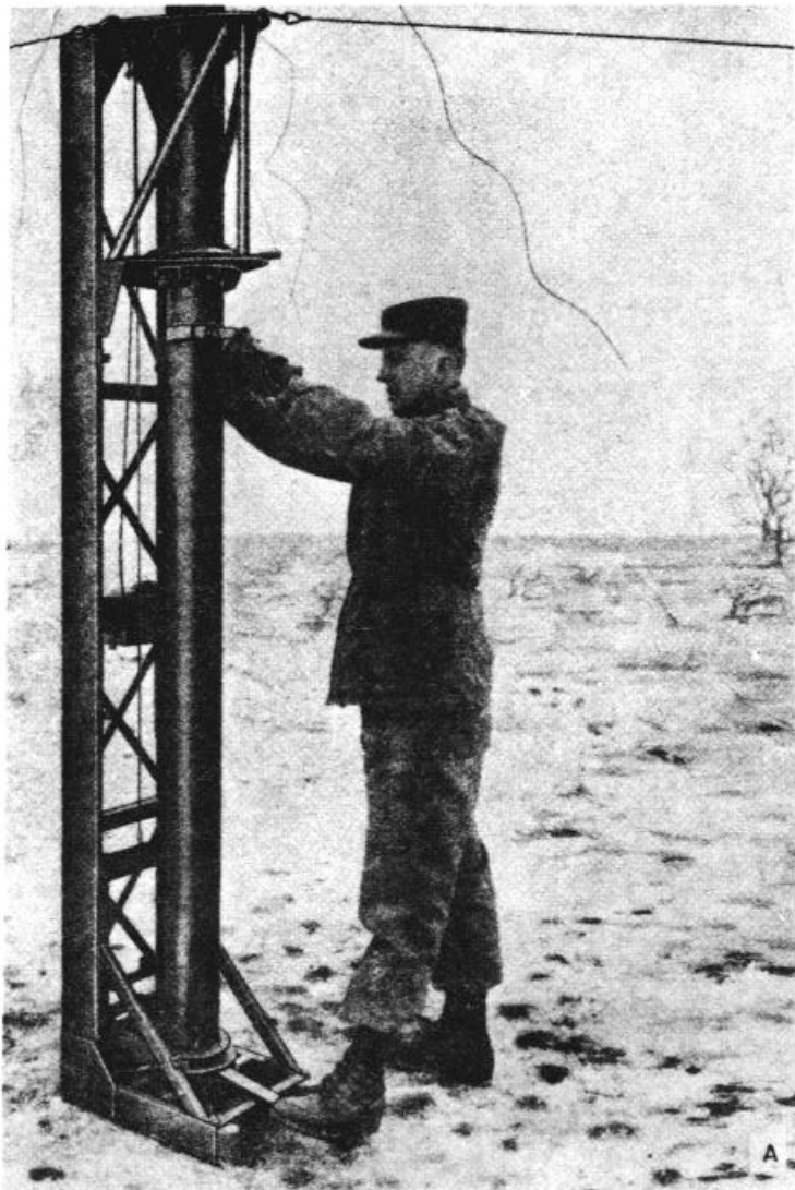
Figure 2-19(2). Raising mast (part 2 of 4).
