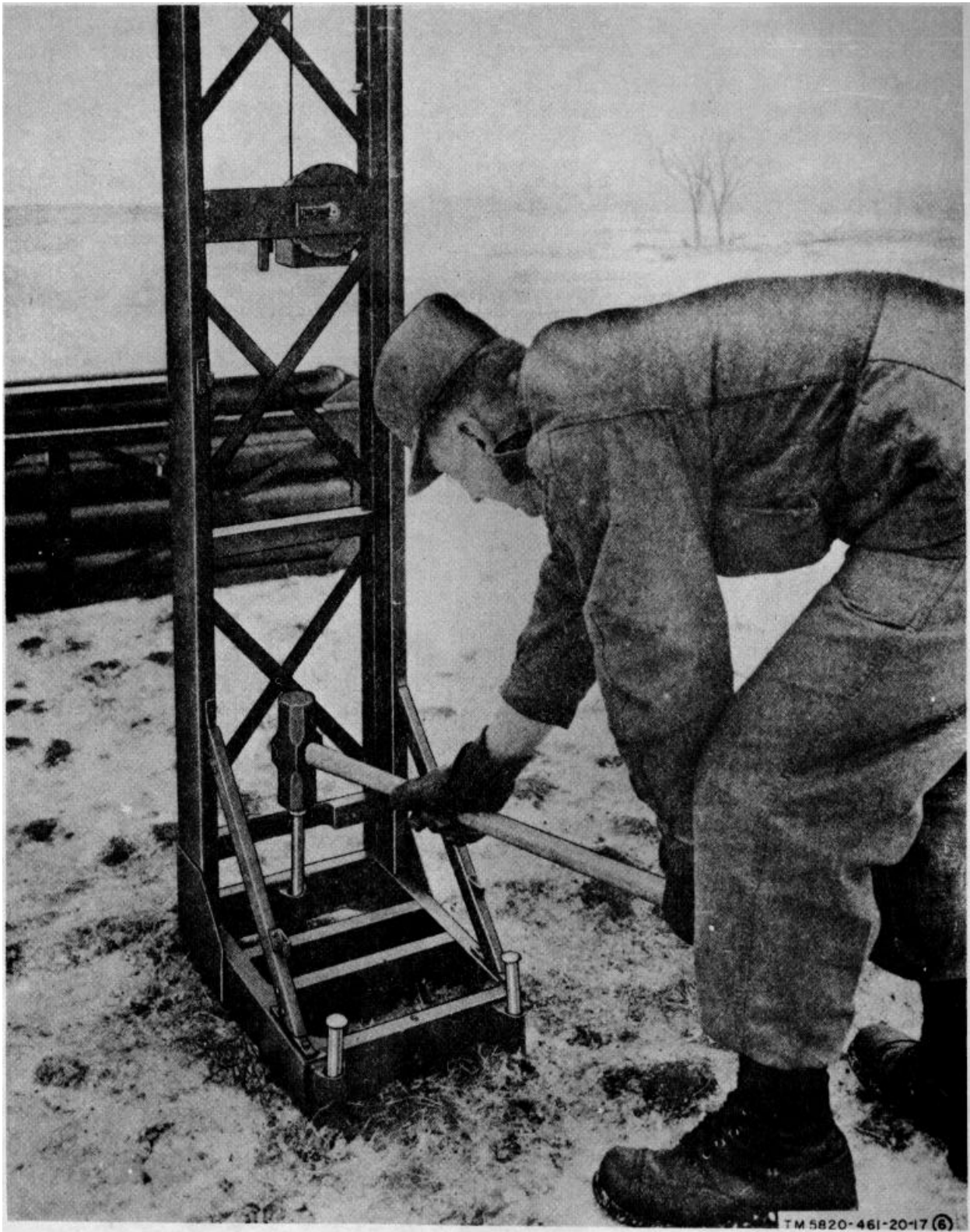
Figure 2-17(6). Erection of launcher (part 6 of 9).
