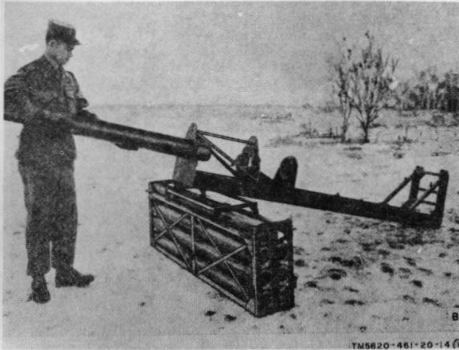
Figure 2-12(1) Antenna mounting procedure (part 1 of 4).
