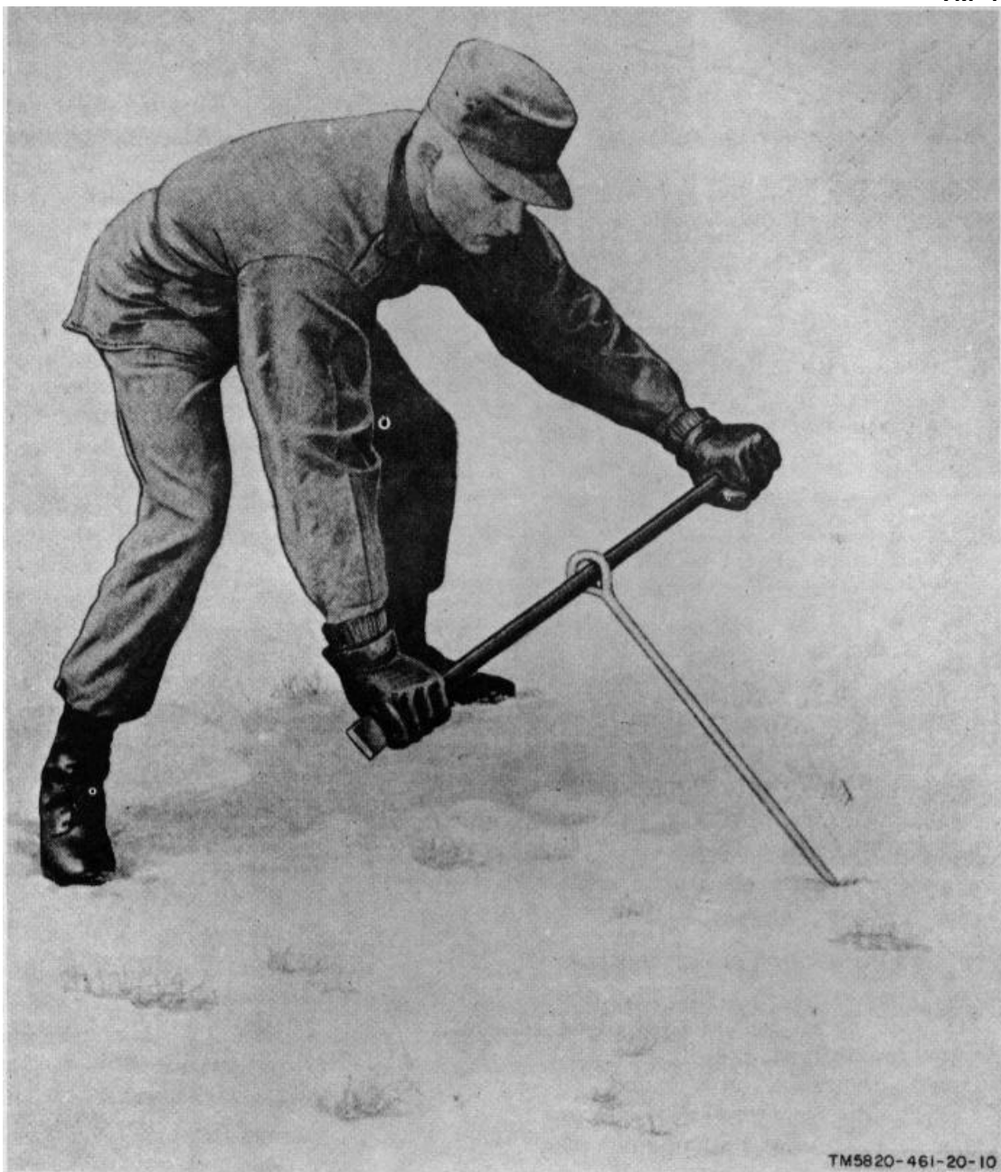
Figure 2-7. Use of digging bar with screw-type guy anchor.
