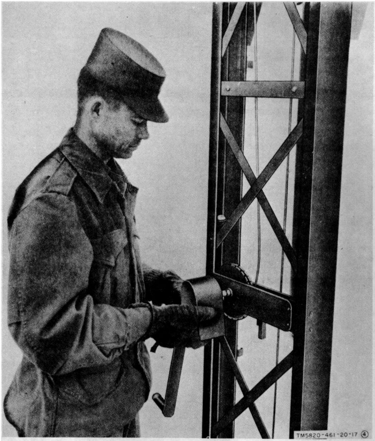
Figure 2-17(4). Erection of launcher (part 4 of 9).
